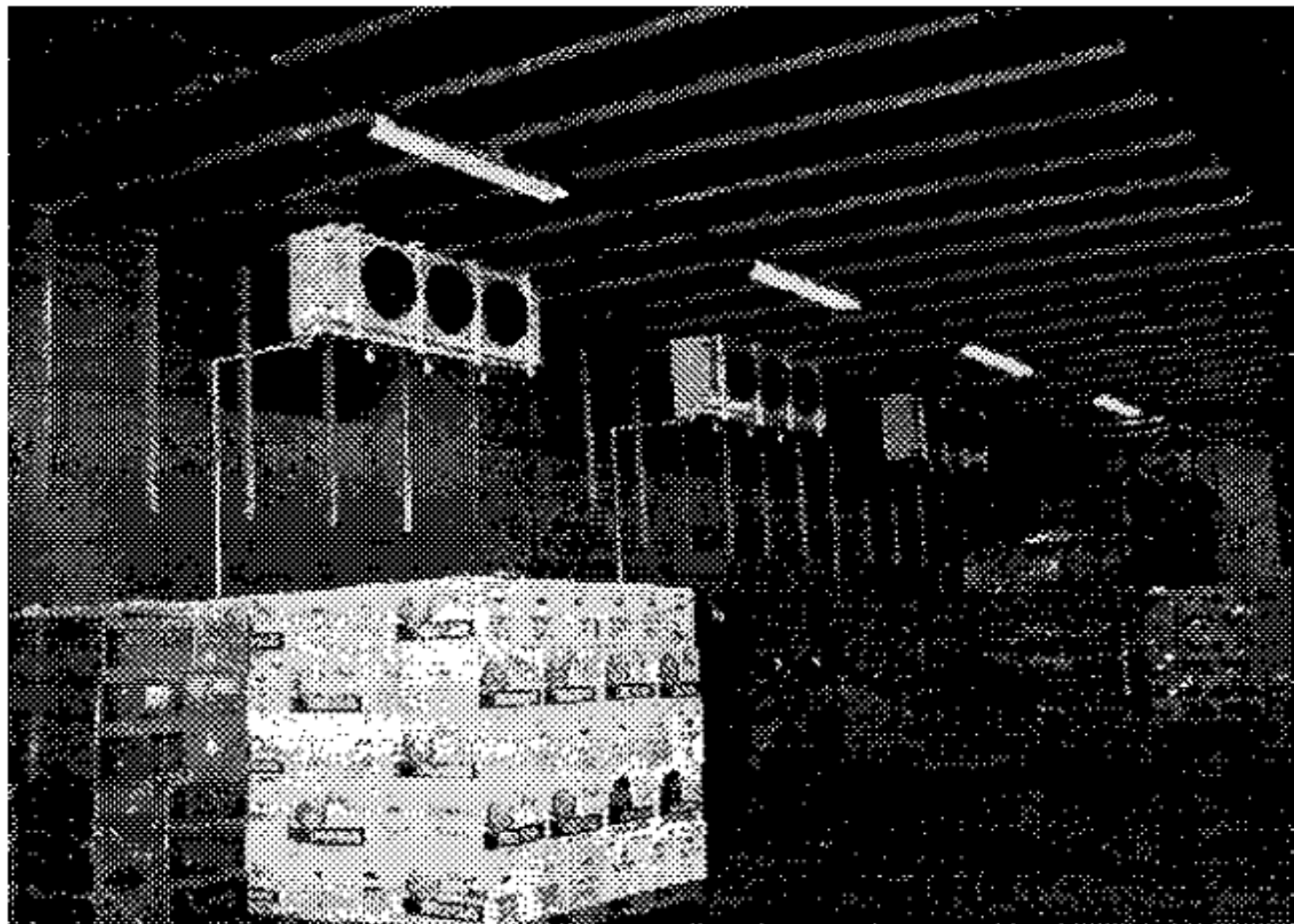
Fig. 6 Refrigerated storage room cooled by mechanical refrigeration.
